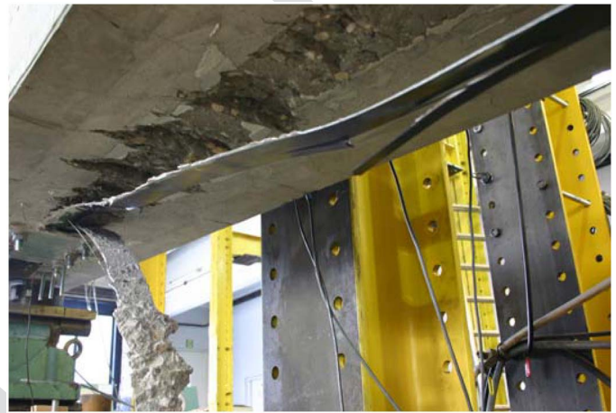
Fig. 5. View of slab after primary failure due to CFRP debonding showing the “fish bone” crack pattern on the bottom of the slab
