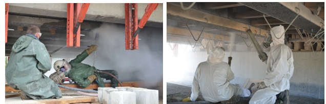
Fig. 12 Girder preparation.
