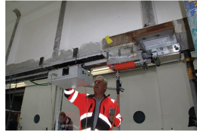
Fig. 6 EB-pCFRP system installation; prestressing rams and heating box shown.
