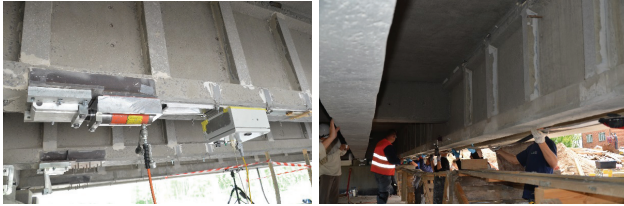
Fig. 13 Flexural strengthening of the bridge girders.
