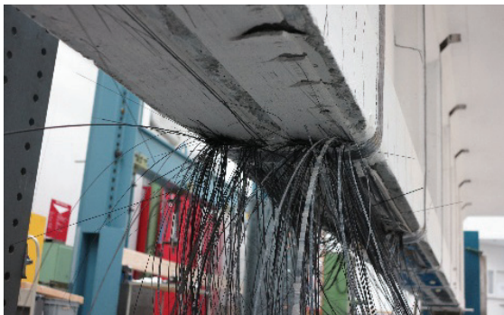
Fig. 9 CFRP rupture of strengthened Girder 2.
