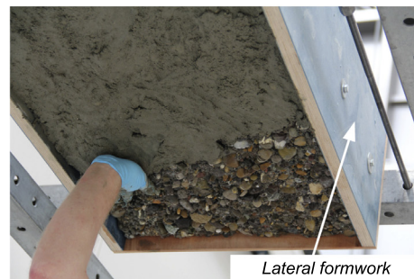
(b) Mortar application at Empa - Investigation 2
