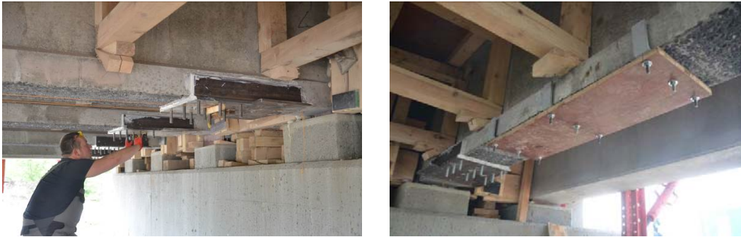
Figure 6. Mounting of steel frames and L-shaped pieces mechanically fastened with bolts.
