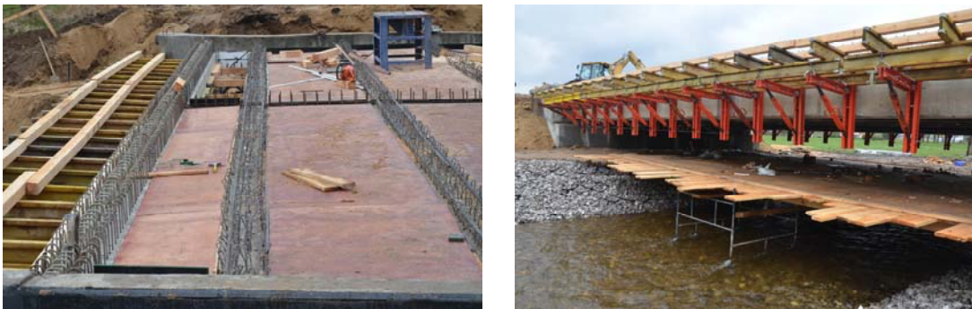
Figure 4. Concrete bridge deck casting (top and side view).
