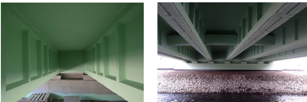
Figure 11. Bridge after strengthening and painting.
