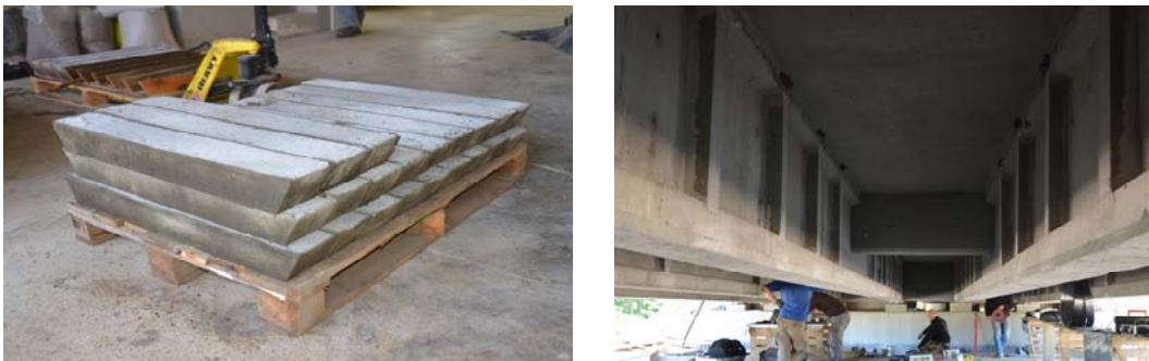
Figure 9. Preparation of concrete trapezoid-shaped filling elements for shear strengthening.
