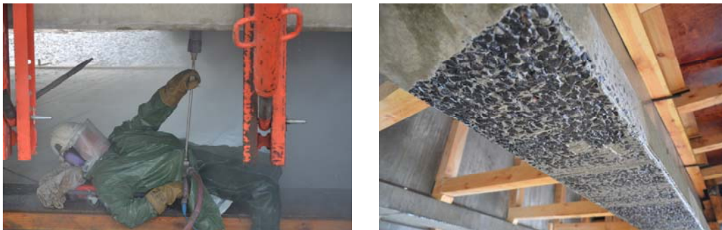
Figure 5. Process of water-jet surface preparation, bottom surface after water-jetting.
