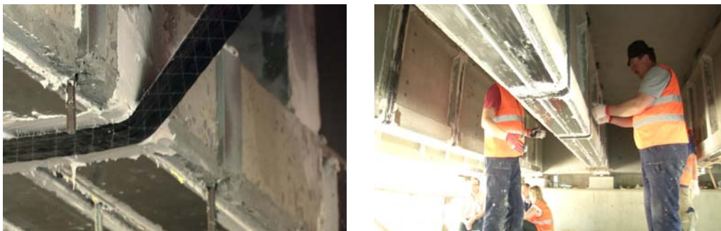
Figure 10. Shear strengthening.
