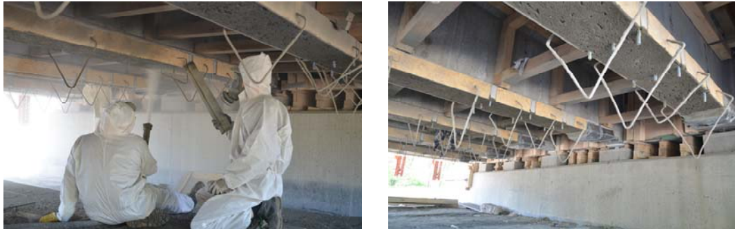
Figure 7. Reprofiling of bridge girders with dry-shotcrete, view the bottom girders.
