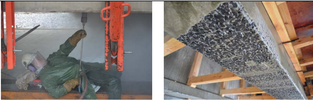
Figure 8. Process of water-jet surface preparation, bottom surface after water-jetting.
