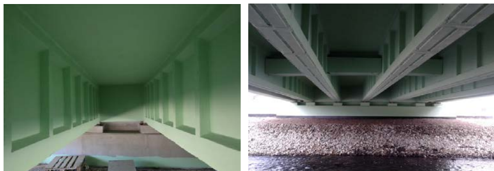
Figure 11. Bridge after reconstruction.
