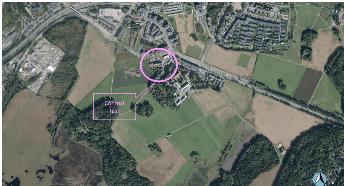
Figure 7. Top aerial view of the project site.
